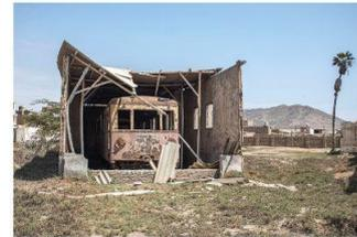
COLAPSO DE LA COBERTURA DE LAMINAS DE ETERNIT EN EL DEPOSITO, AFECTANDO A LA INFRAESTRUCTURA QUE LA SOSTIENE Y A LA LOCOMOTORA QUE ALBERGA
