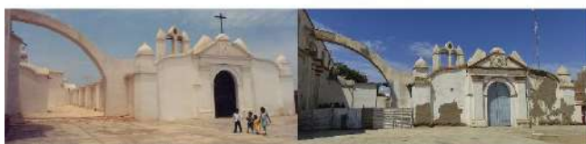
Fachada principal de "La Ramada"
