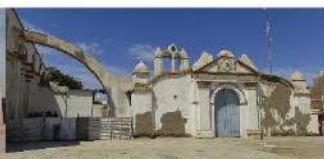
Fachada principal de "La Ramada" 2021
